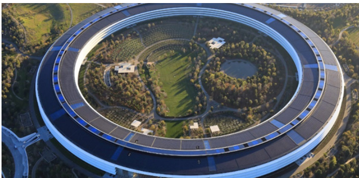
Apple's building in California isolated using sliding bearings (source: New York Times)
