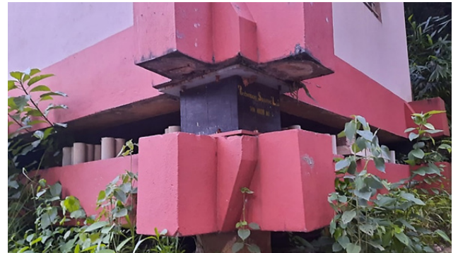
A building at IIT Guwahati campus isolated using rubber bearing
